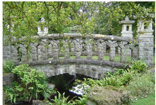
The Japanese Bridge
